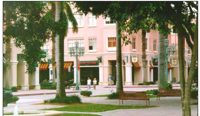
The character of the ground floor commercial frontage in this mixed use center is determined by the continuous arcades running along both sides of a long square. The dimensions, form, and spacing of the arcade piers are quite consistent.
