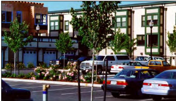
Interior-of-Block parking, often shared by both residential and commercial uses, may be built as structured parking or (for the short term) surface parking.
