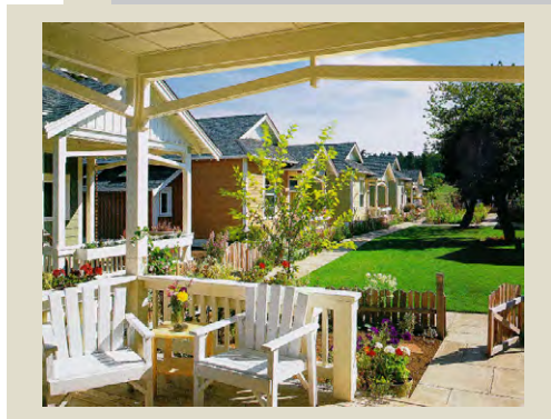
Green Court Cottages
