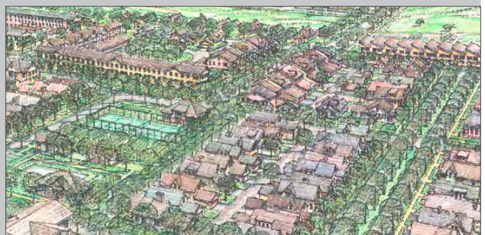
View of Single Family Houses in Eagle Village
