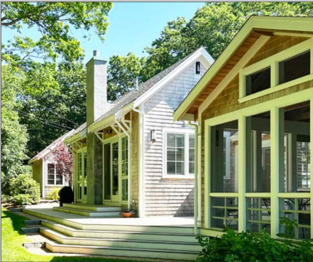
Deck between Bedroom and Porch
