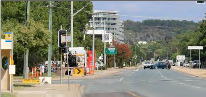
EXISTING CONDITION REPRESENTATIVE SETTING
